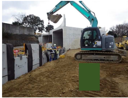
壁面材組立て
