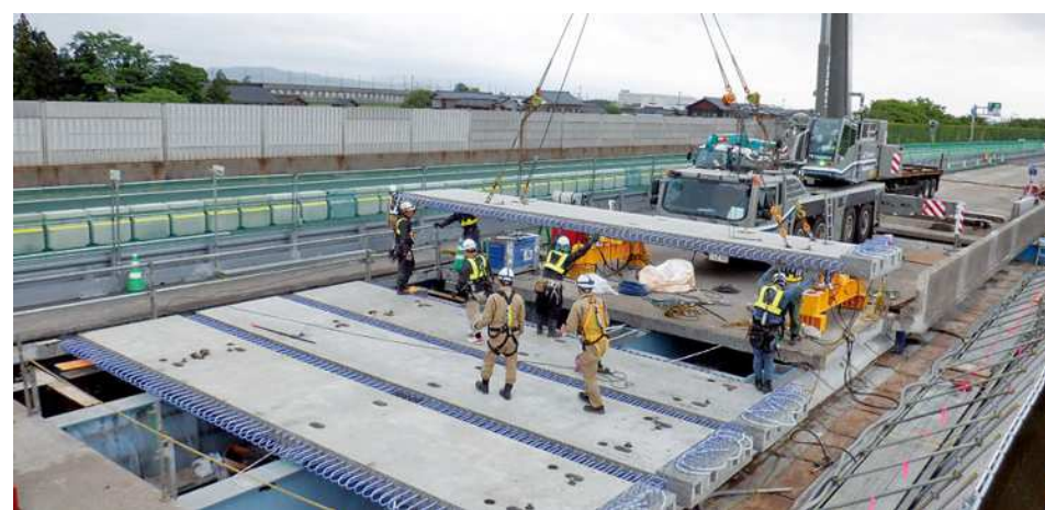
橋梁の床版取替
