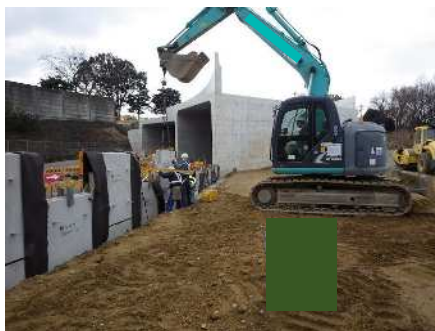
壁面材組立て
