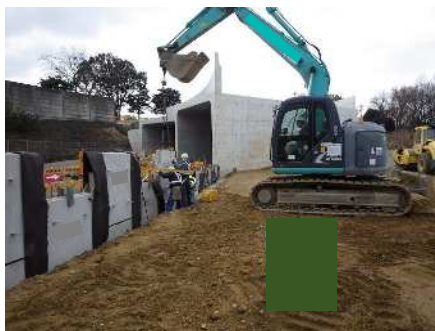
壁面材組立て
