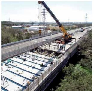
Replacing bridge deck slabs
