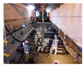
Installing inverted arches of a tunnel
