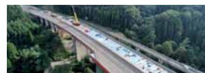
Example of bridge deck slab replacement work
