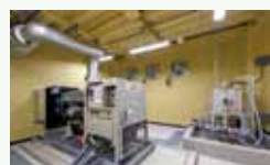
Installation of power generator for power outages
