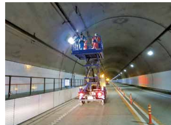
Inspection of tunnel lighting
