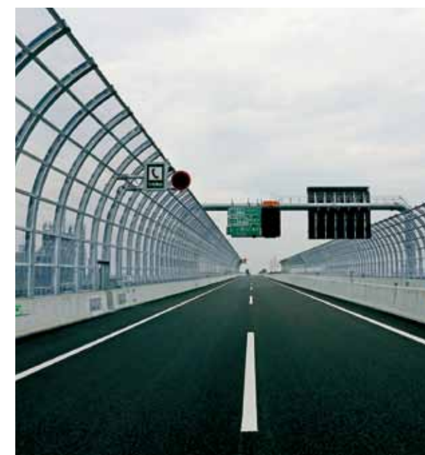
Noise barriers installed on the Gaikan Expressway (between Misato-Minami IC and Koya JCT)
