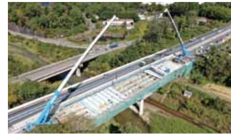
Replacing bridge deck slabs
