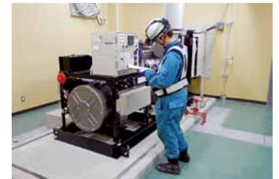
Inspection of power generator
