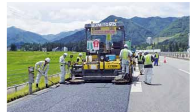
Repairing pavements
