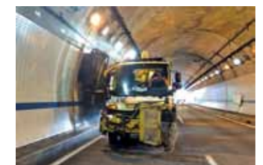
Cleaning walls of the tunnel
