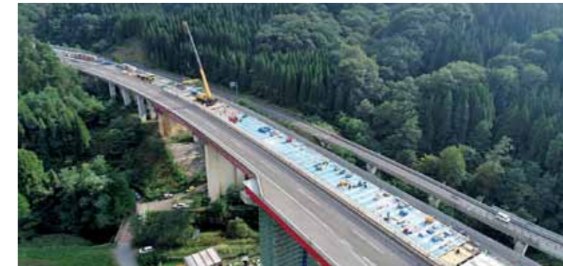
Example of bridge deck slab replacement work
