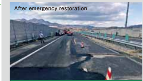
The emergency restoration was completed within approximately 16 hours after the disaster.
