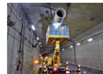
Cleaning ventilation tunnel
