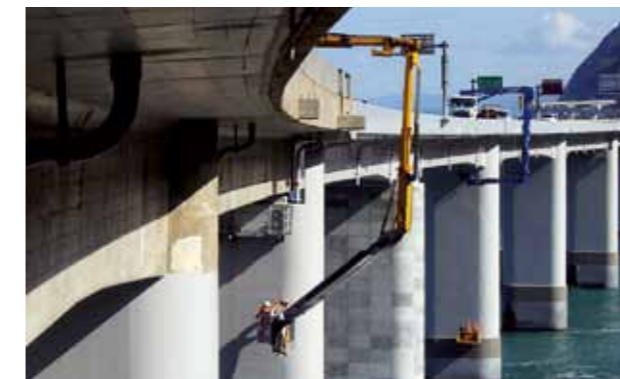
Inspecting the bridge
