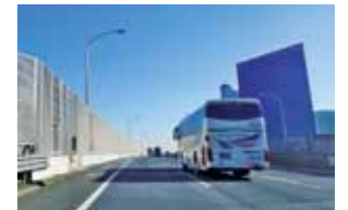
Example of Noise barriers installed
