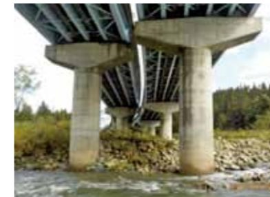
Before pier reinforcement
