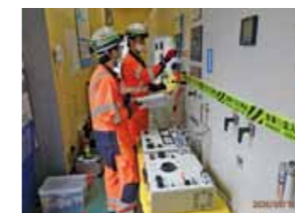
Inspecting the power receiving and distribution equipment
