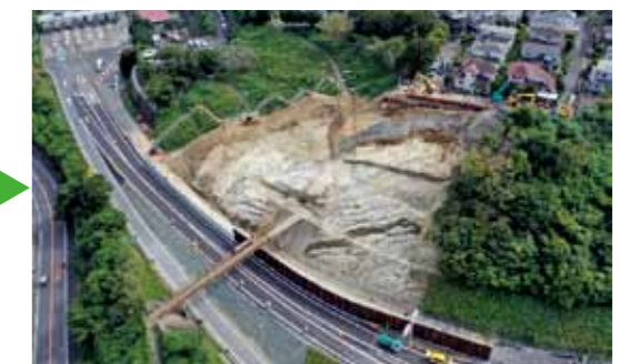
Zushi IC on the Yokohama-Yokosuka Expressway after the cut slope failure caused by heavy rain (left) and after resuming service (right)
