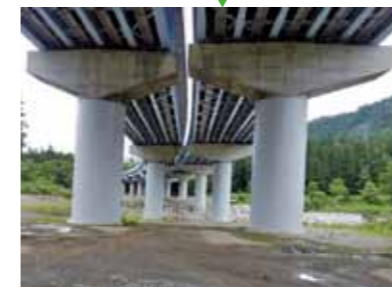
After pier reinforcement
