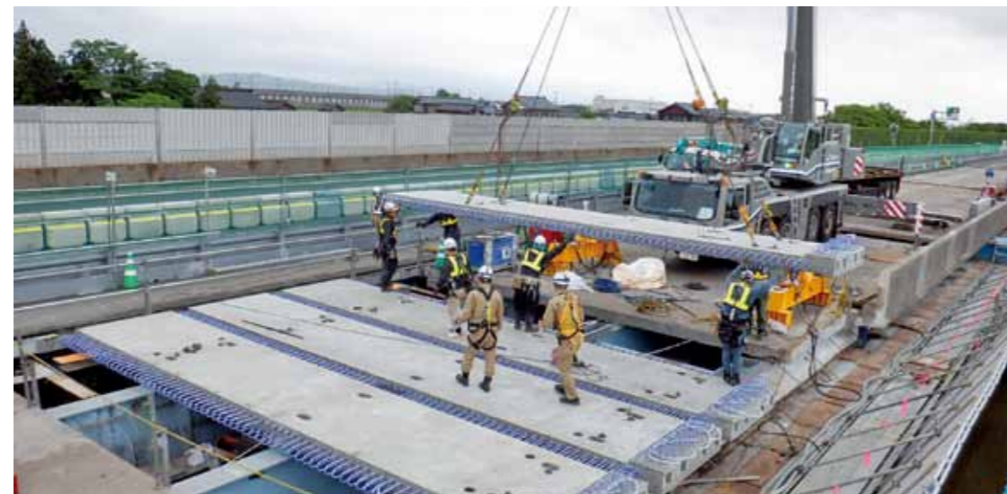
橋梁の床版取替
