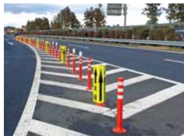
Countermeasures for wrong-way driving at a ramp merging section
