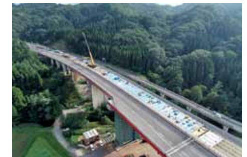
Example of bridge deck slab replacement work
