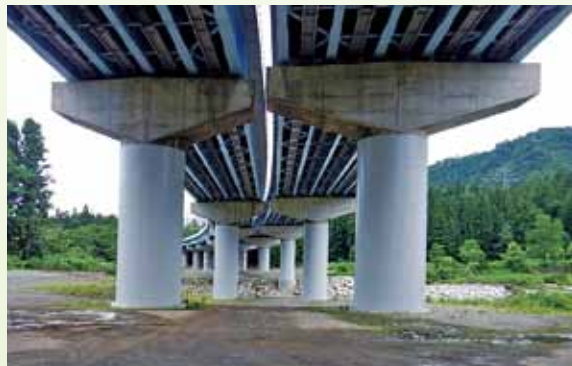
Example of pier reinforcement (steel jacketing) work
