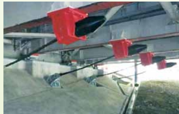
Example of bridge collapse prevention device installation
