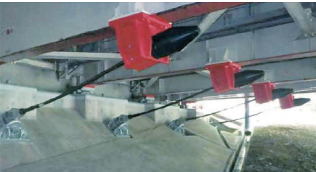
Example of a bridge collapse prevention device
