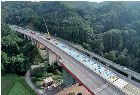
Example of bridge deck slab replacement work
