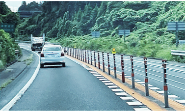
Lane departure prevention (Cable barriers installed in the provisional two-lane section)
