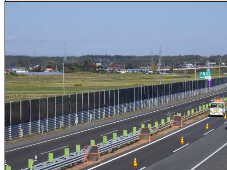
新設防雪柵 H=4.0m
