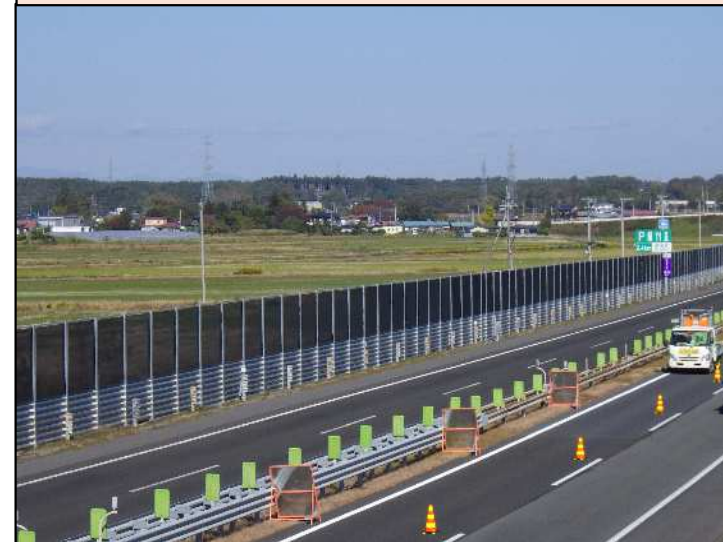
新設防雪柵 H=4.0m
