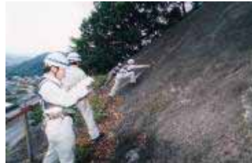
(のり面の点検)
