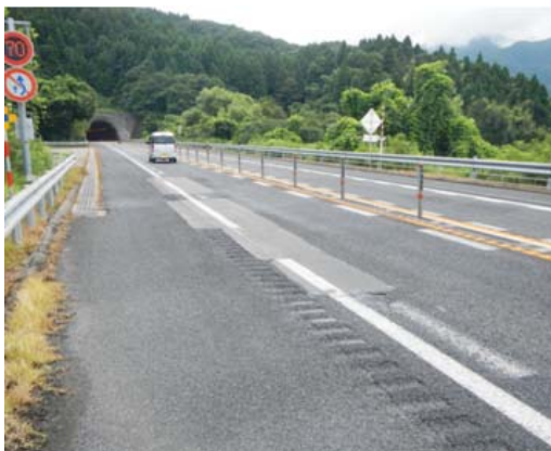
舗装路面の補修(三川IC～安田IC間)
